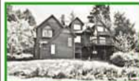
132 SHELIKOF ST.— Recent foundation upgrades! $449,500
